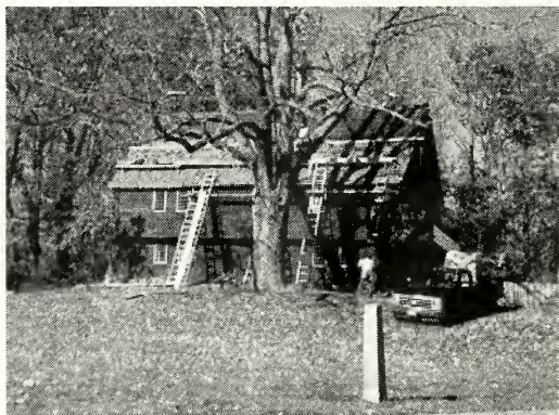
Replacing the Capen House roof
